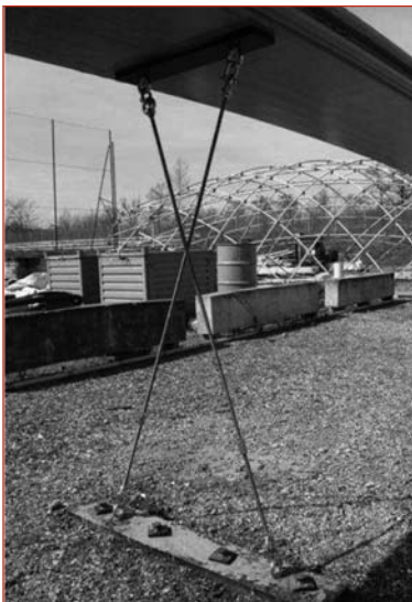
Figure 13 : Appui central croisé.
